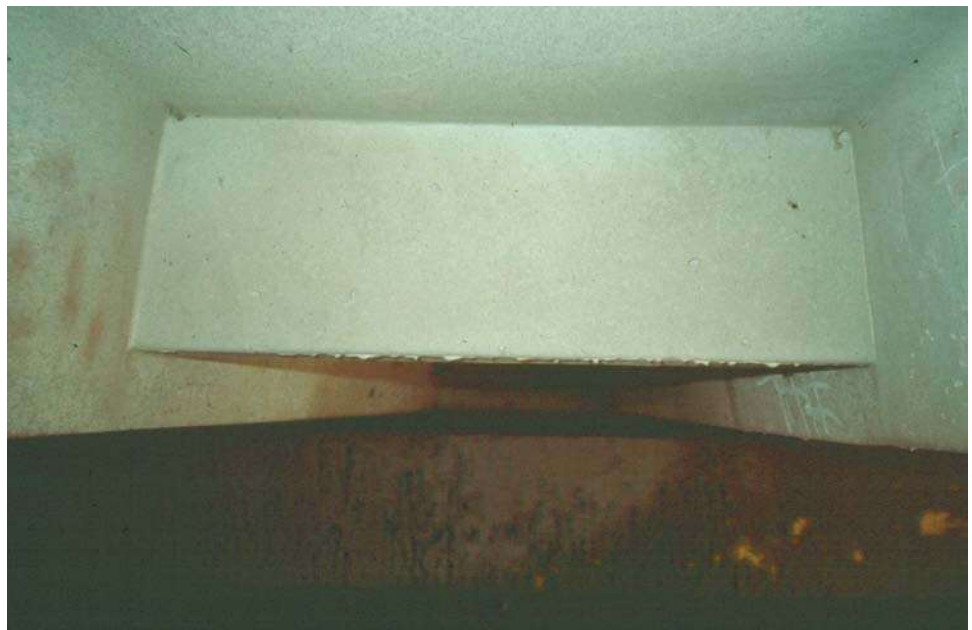
Figure 9.4.9 Close-up of Intermediate Diaphragm
