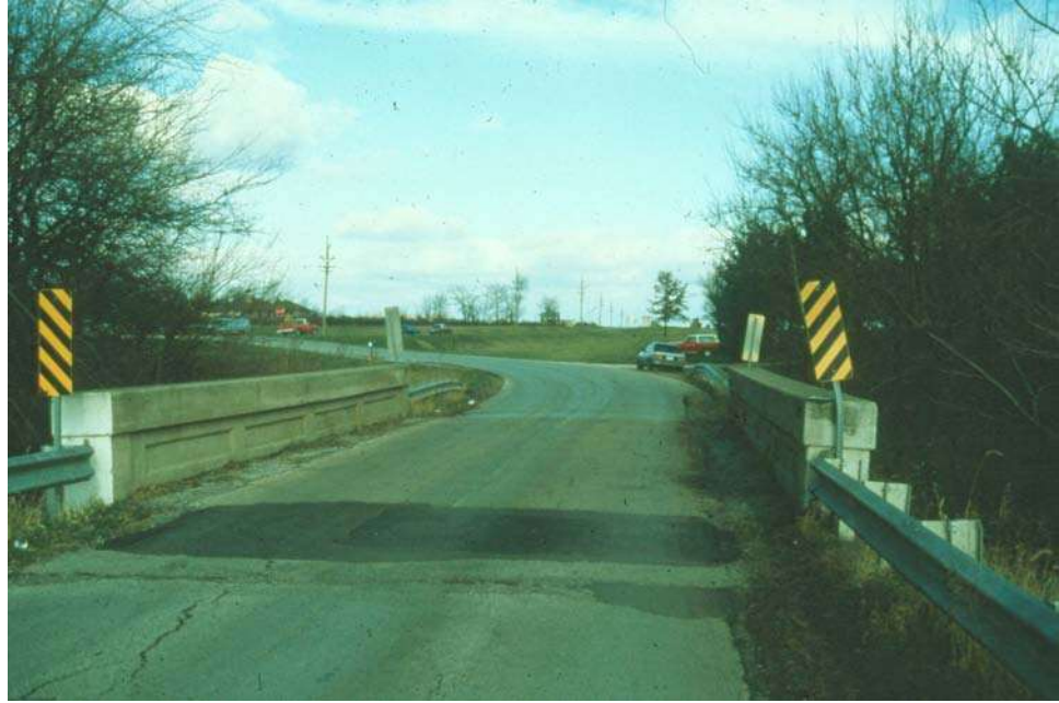
Figure 9.3.2 Concrete Through Two-Girder Bridge
