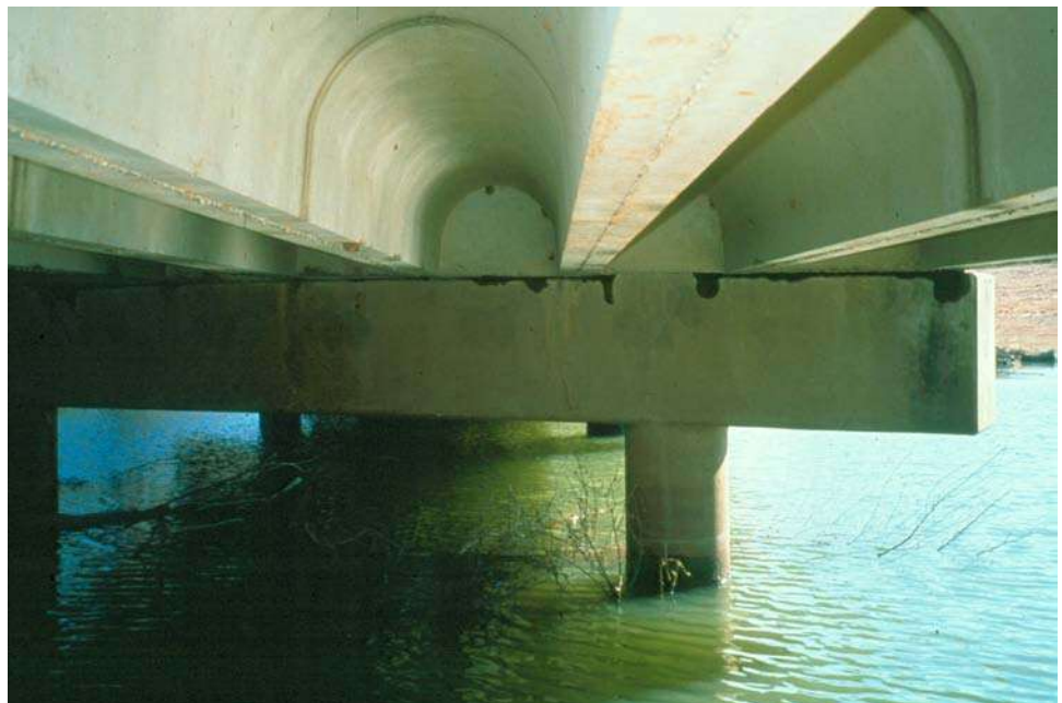
Figure 9.4.2 Underside View of a Cast-in-Place Channel Beam Bridge
