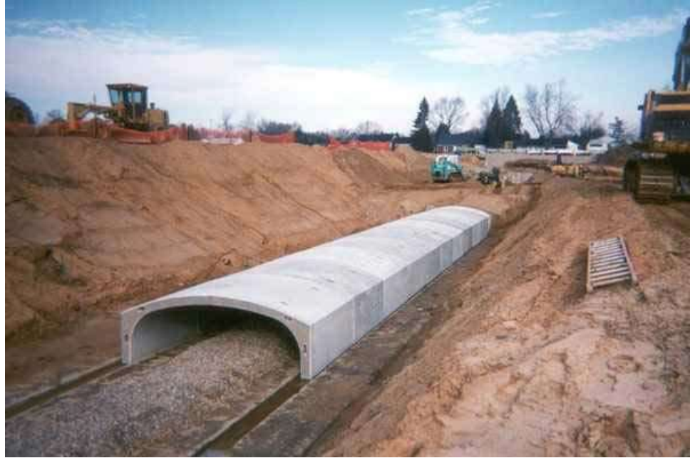
Figure 9.5.4 Precast Concrete Arch with Integral Vertical Legs
