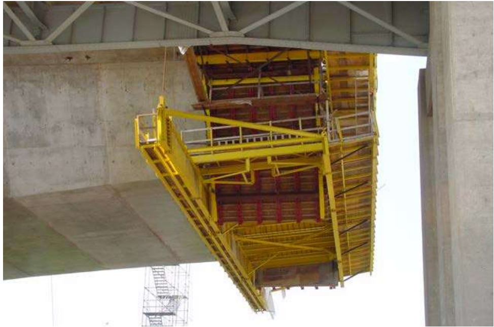
Figure 9.11.17 Cast-in-place Box Girder Segment
