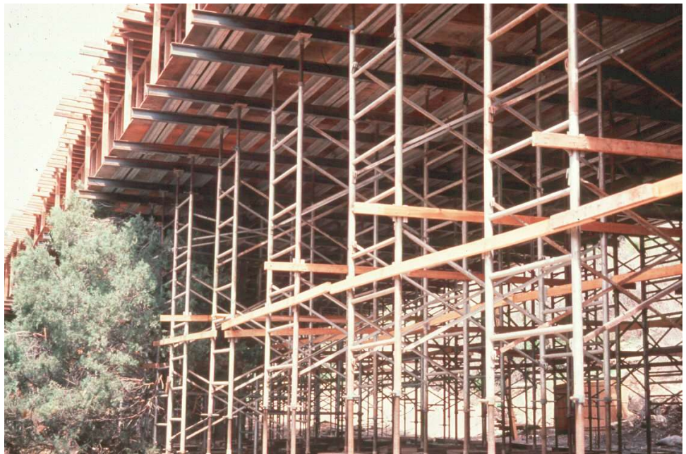
Figure 9.11.5 High Level Casting Formwork on Falsework
