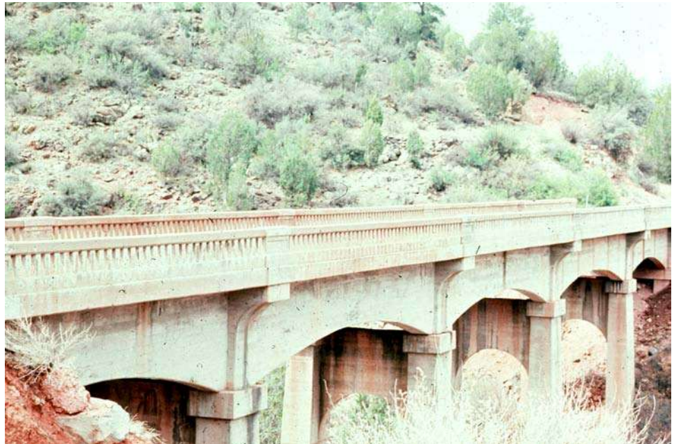
Figure 9.3.1 Concrete Deck Two-Girder Bridge
