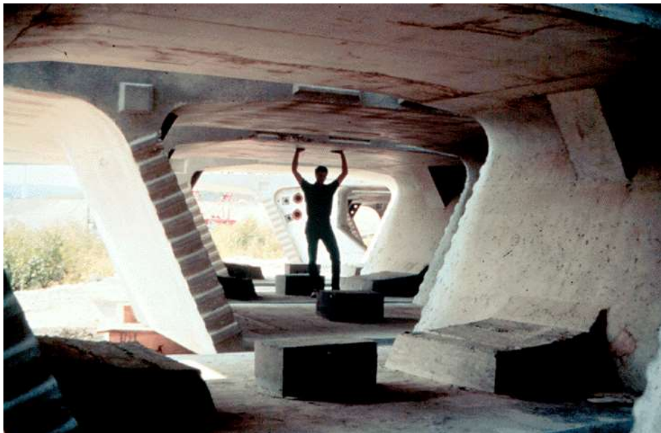
Figure 9.11.16 Box Girder Segment
