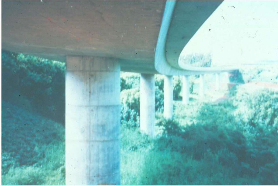
Figure 9.11.2 Cast-in-place Concrete Box Girder Bridge
