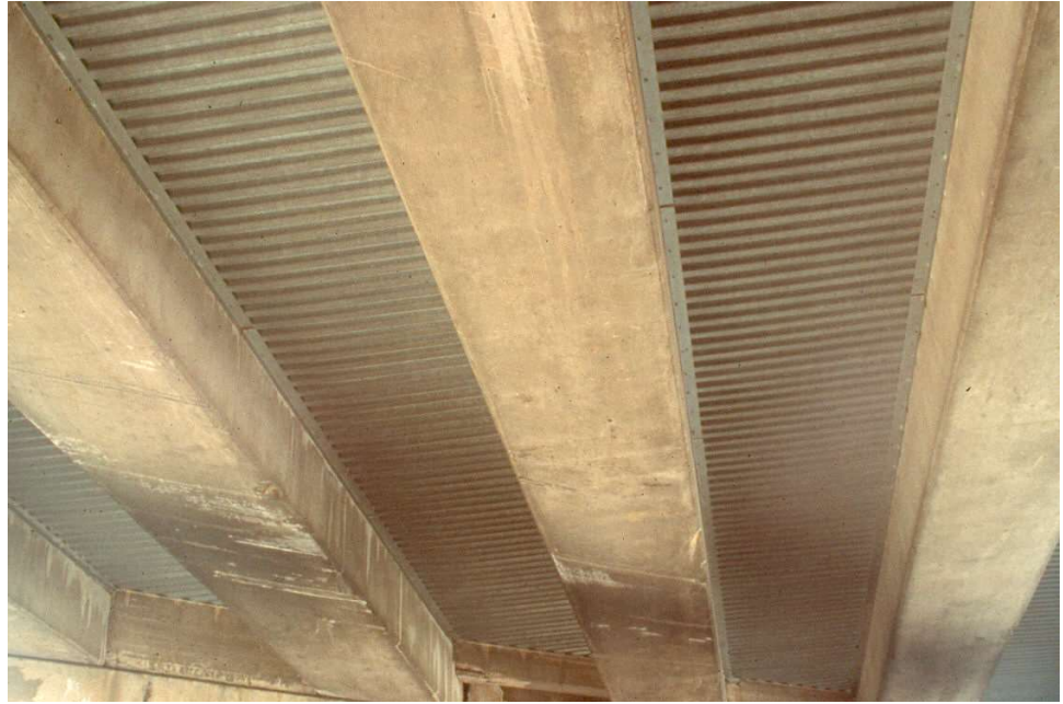
Figure 9.10.7 Underside of a Typical Spread Box Beam
