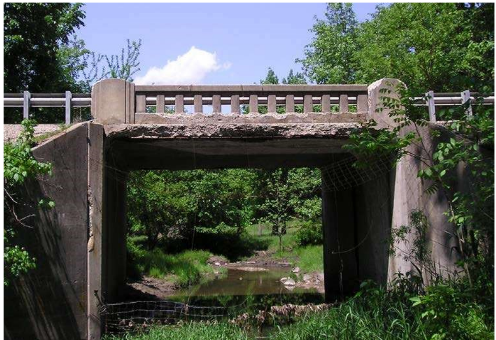
Figure 9.1.1 Typical Simple Span Cast-in-Place Slab Bridge
