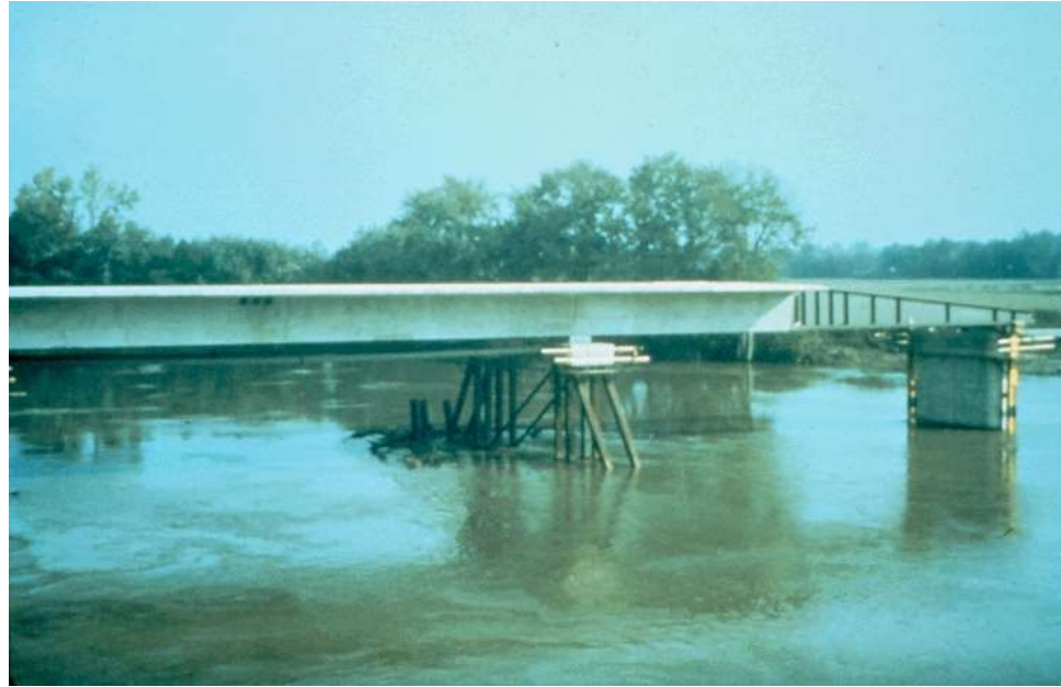
Figure 9.11.27 Incremental Launching Overview (Note Temporary Pile Bent)
