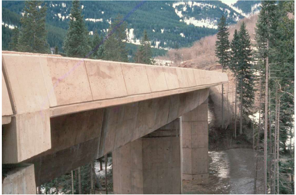
Figure 9.11.4 Cast-in-place Concrete Box Girder Bridge
