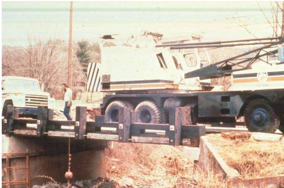
Figure 8.3.3 Stress-Laminated Timber Slab Bridge
