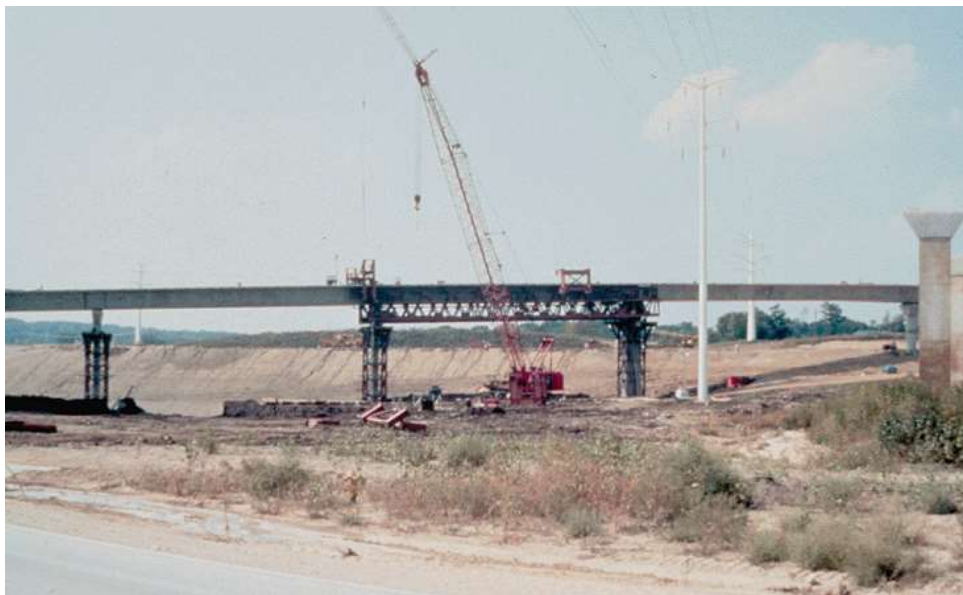
Figure 9.11.23 Span-by-span Construction (with Erection Truss)
