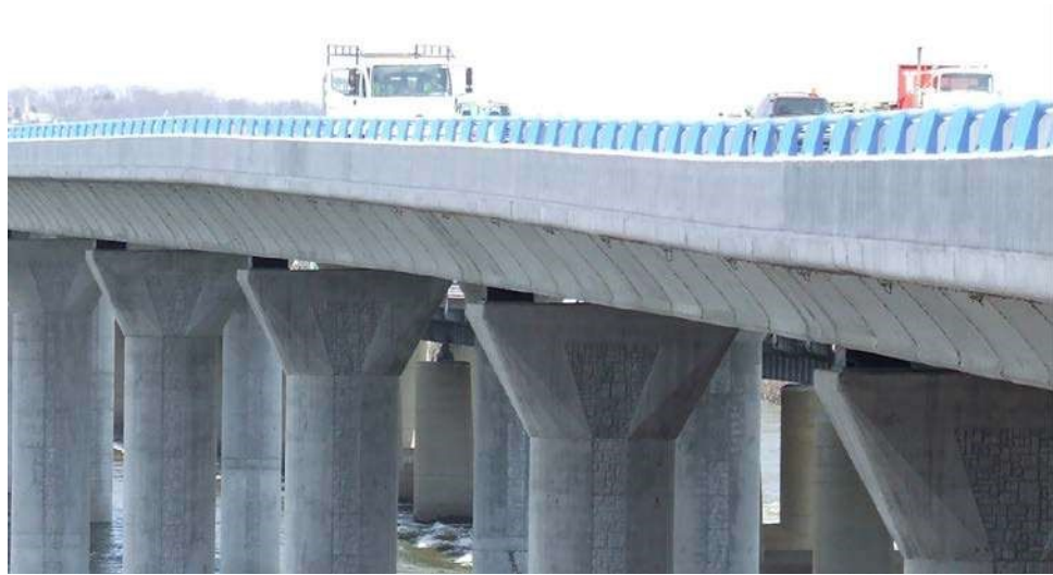
Figure 9.11.14 Segmental Concrete Bridge
