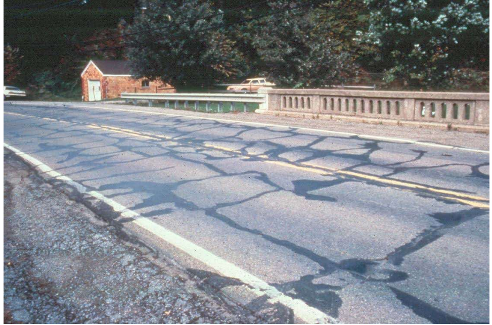
Figure 9.2.17 Asphalt Covered Tee Beam Deck
