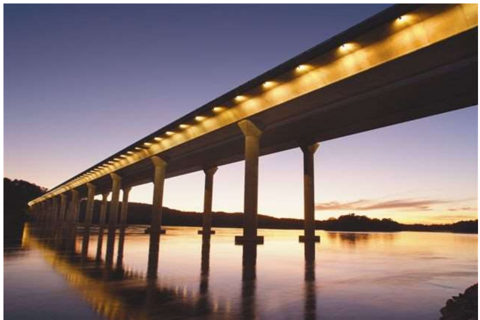
Figure 9.11.1 Segmental Precast Concrete Box Girder Bridge
