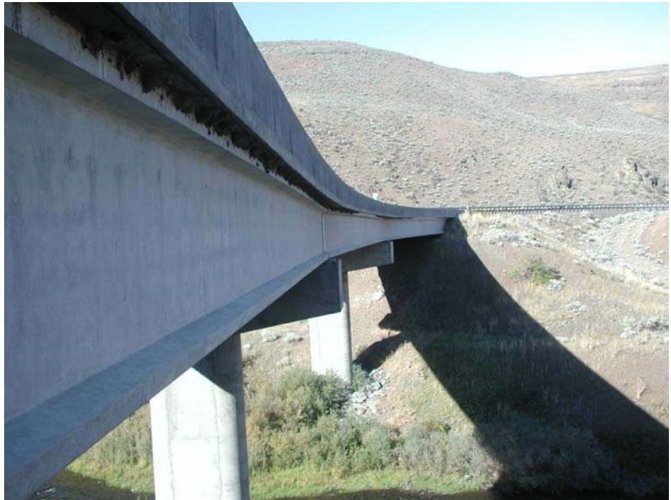
Figure 9.9.1 Prestressed I-beam Superstructure
