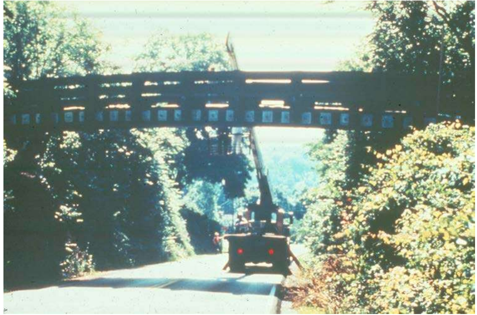
Figure 8.3.4 Glulam Stress-Laminated Timber Slab Bridge
