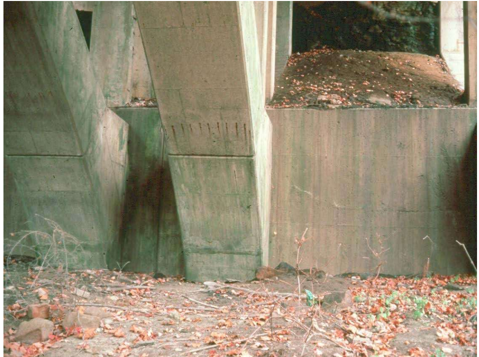
Figure 9.5.12 Arch/Skewback Interface
