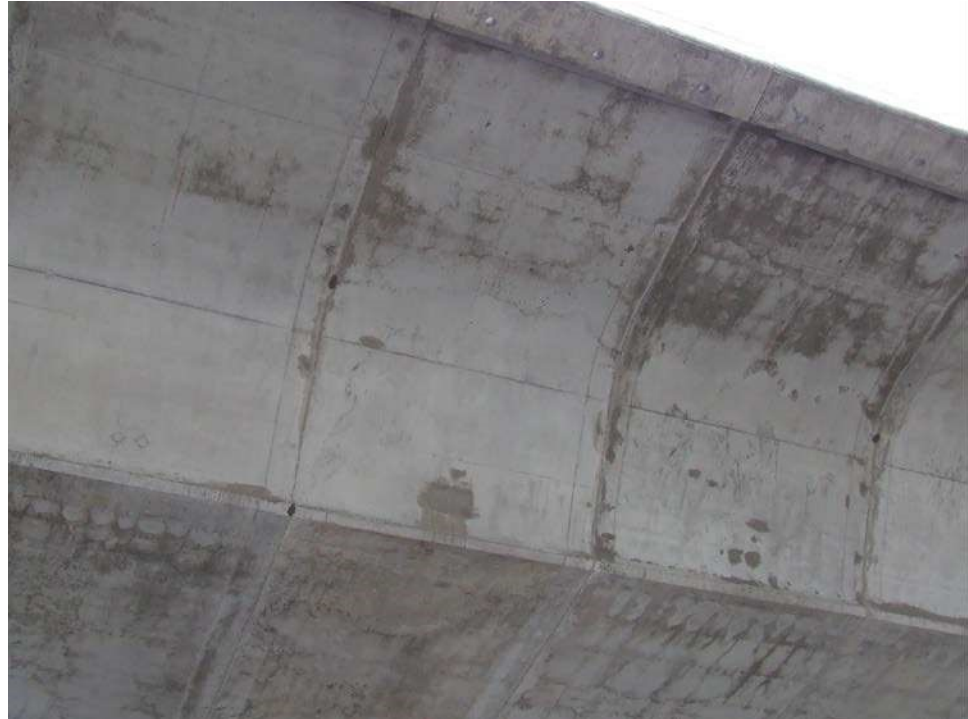
Figure 9.11.15 Close-up of Box Girder Segments
