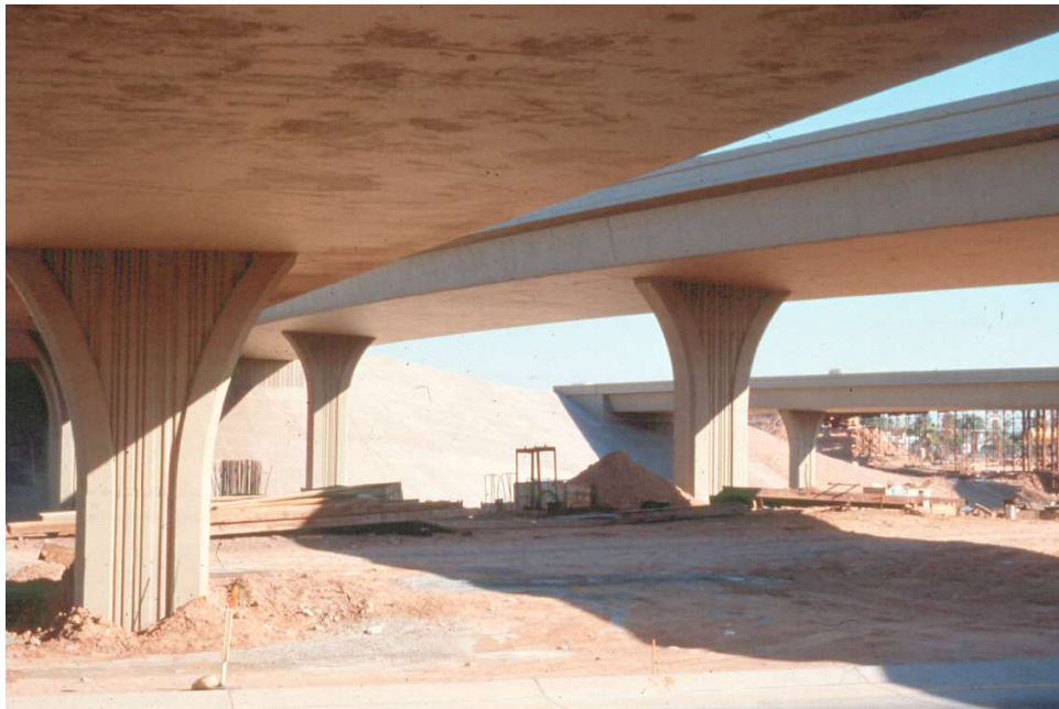
Figure 9.11.7 At-grade Casting – After Supporting Earth Removed
