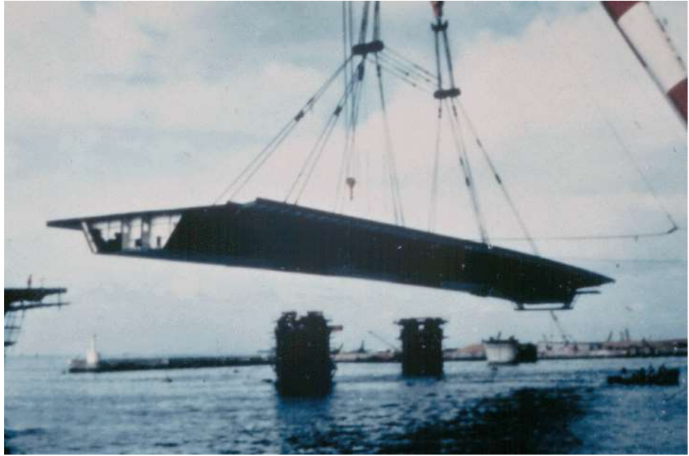
Figure 9.11.24 Span-by-span Total Span Erection (Lifting)
