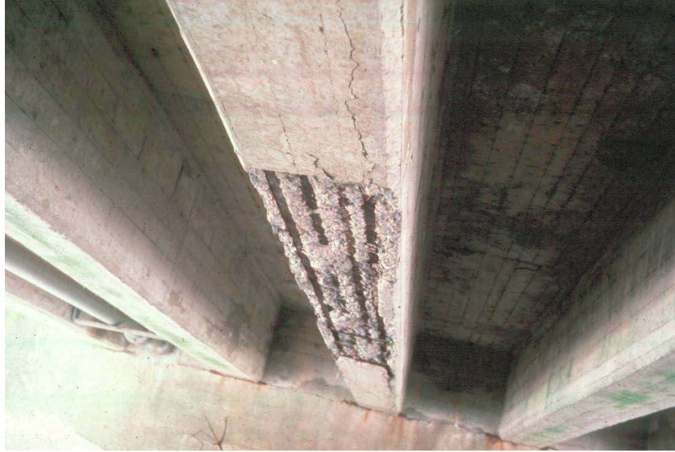
Figure 9.2.16 Spall on the Bottom of the Stem of a Tee Beam with Corroded Main Steel Exposed
