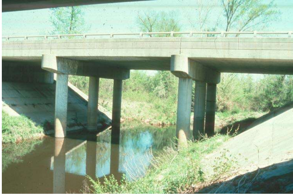
Figure 9.1.2 Typical Multi-Span Cast-in-Place Slab Bridge
