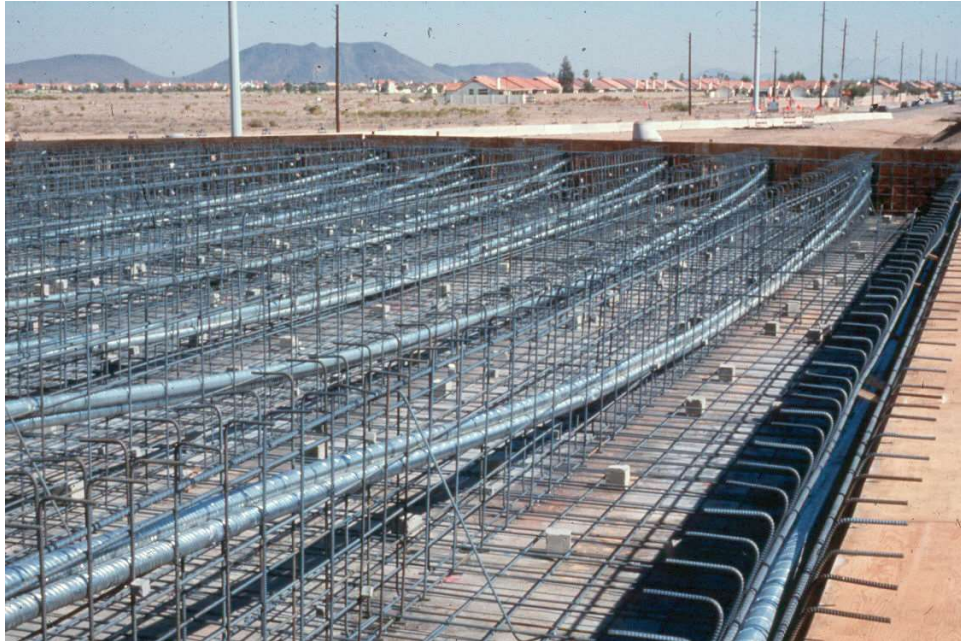
Figure 9.11.6 At-grade Formwork with Post-tensioning Ducts
