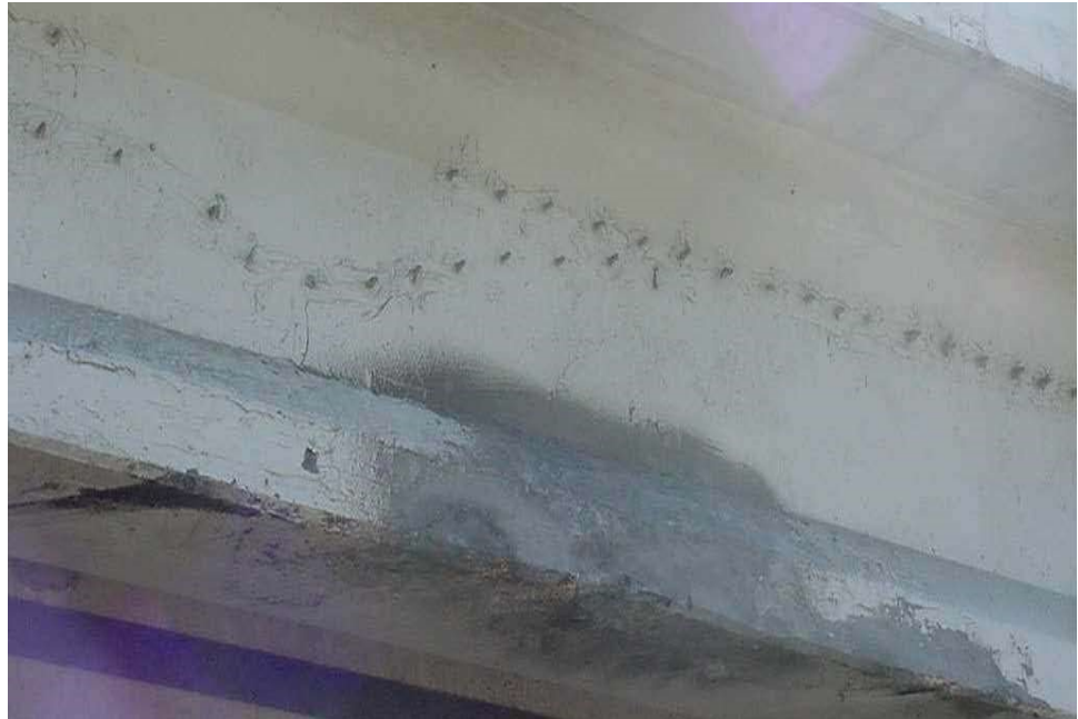
Figure 9.9.21 Collision Damage Repair on Prestressed Concrete I-Beam. Note Epoxy Injection Ports and Guniting Repair
