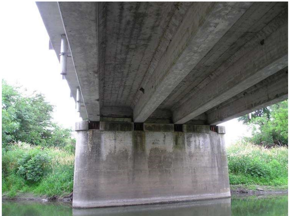
Figure 9.2.1 Simple Span Tee Beam Bridge
