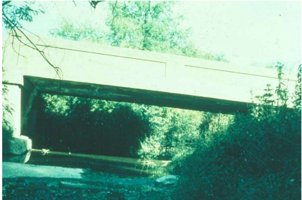
Figure 9.3.4 Concrete Through Two-Girder Elevation View
