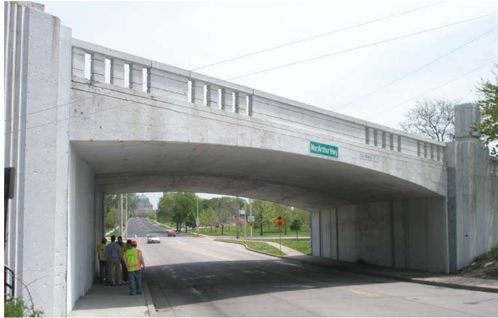
Figure 9.6.2 Single-span Rectangular Concrete Rigid Frame Bridge
