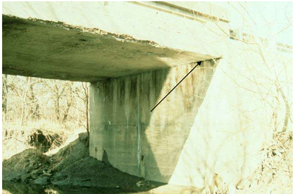
Figure 9.3.6 Bearing Area of a Through Two-Girder Bridge
