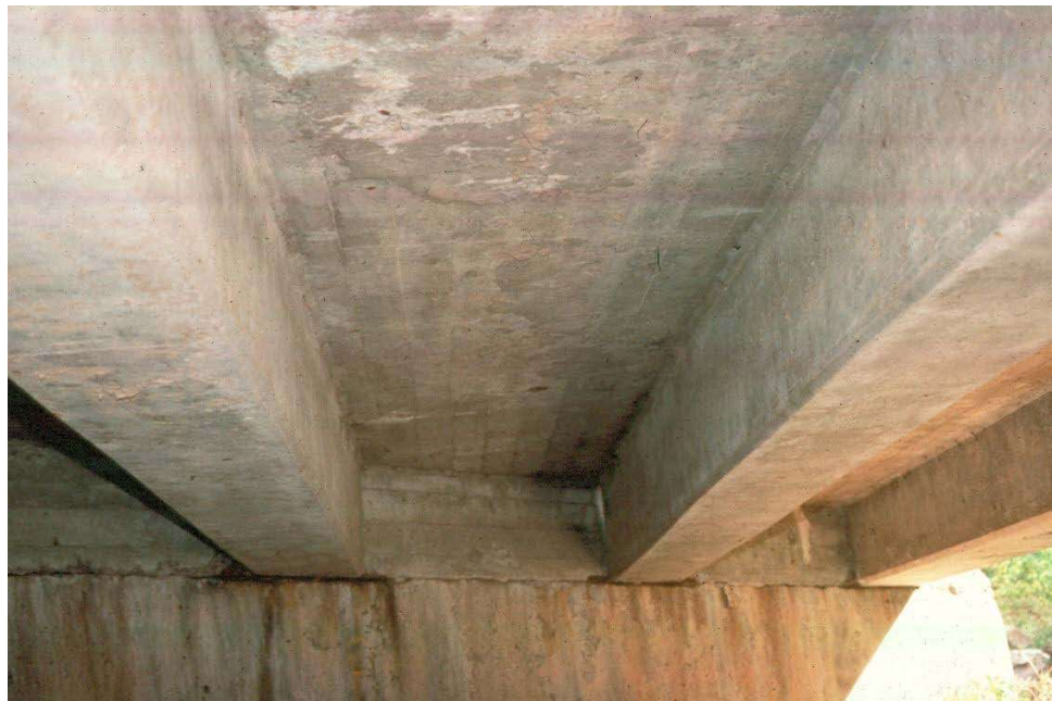
Figure 9.2.3 Typical Tee Beam Layout
