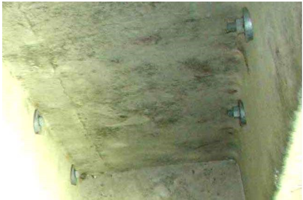
Figure 9.4.7 Stem Tie-Bolts
