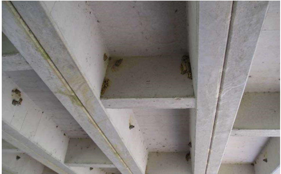
Figure 9.4.1 Underside View of Precast Channel Beam Bridge
