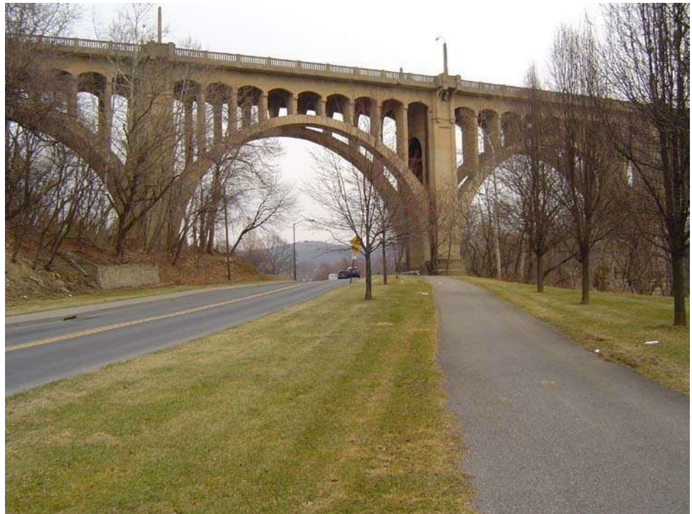
Figure 9.5.1 Open Spandrel Arch Bridge
