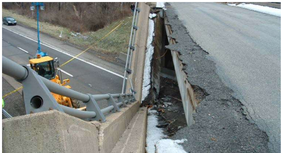
Figure 9.10.21 View East (Ahead Segments) from SR1014 Above Pier 2
