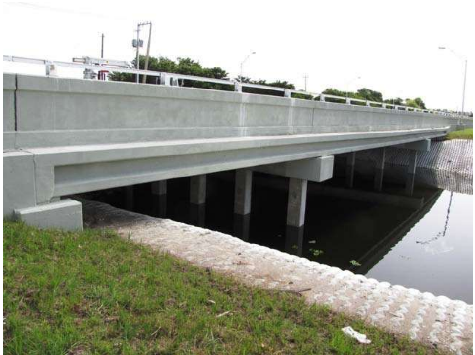
Figure 9.7.3 Poutre Dalle Precast Slab Bridge
