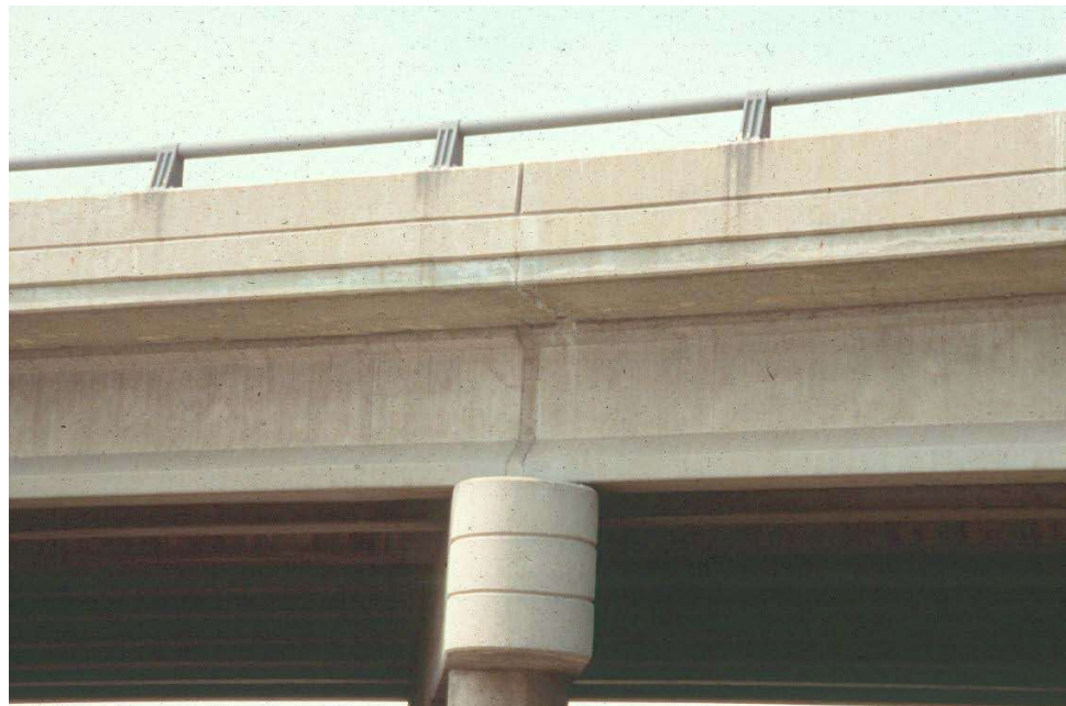
Figure 9.9.9 Continuous Prestressed I-Beam Bridge
