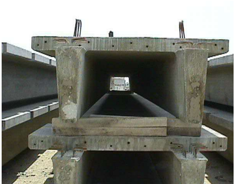
Figure 9.8.1 Typical Prestressed Double Tee Beam
