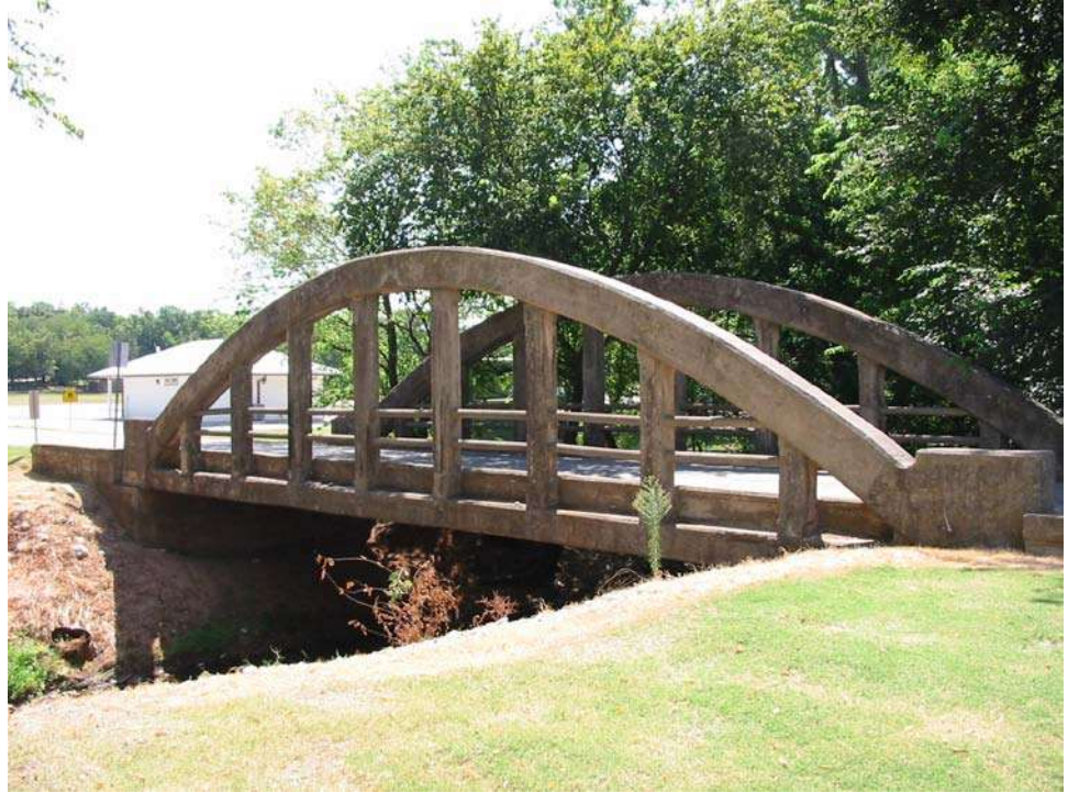
Figure 9.5.3 Concrete Through Arch Bridge
