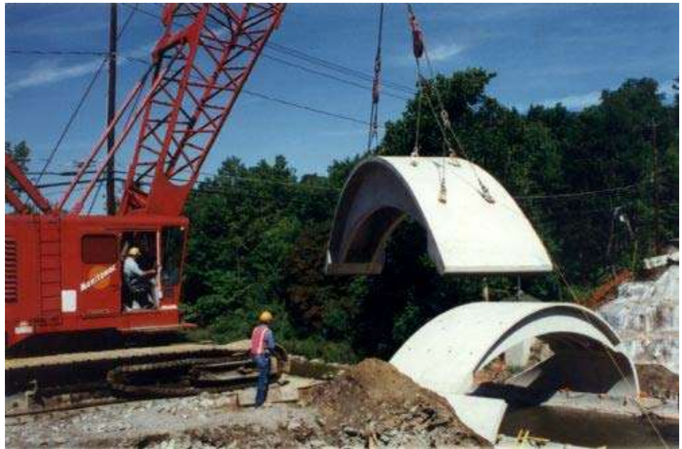
Figure 9.5.5 Precast Segmental Concrete Arch
