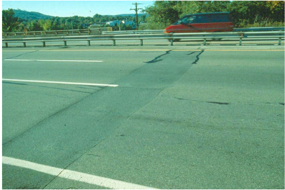
Figure 9.6.13 Roadway of a Rigid Frame Bridge with Asphalt Wearing Surface
