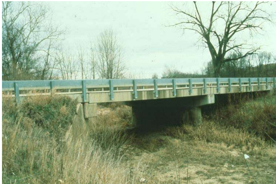
Figure 9.4.3 General View of a Precast Channel Beam Bridge
