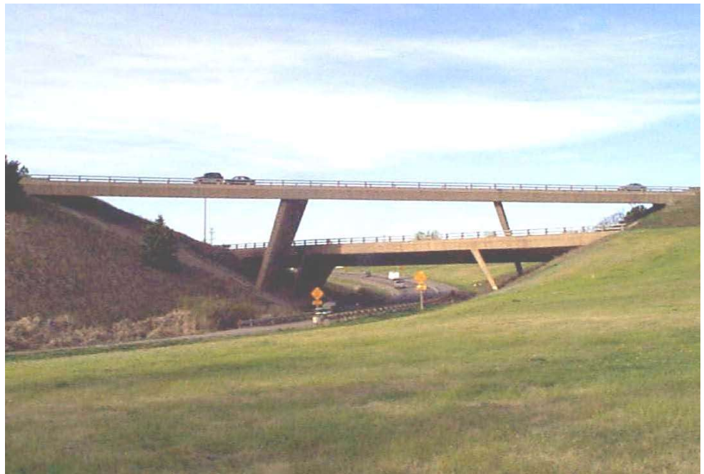
Figure 9.6.1 Multi-span Concrete Rigid Frame Bridges
