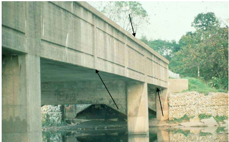
Figure 9.3.7 Typical Elevation View of a Through Two-Girder Bridge with Tension Zones Indicated
