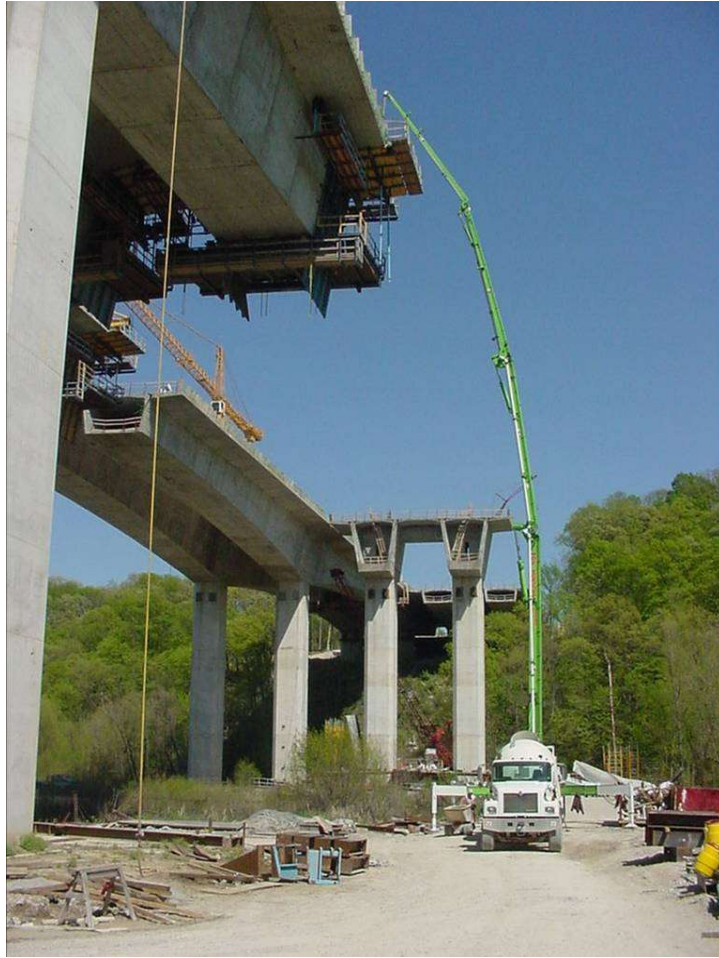
Figure 9.11.25 Progressive Placement Construction
