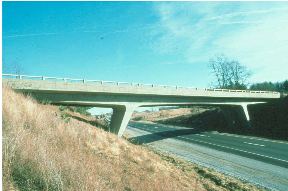
Figure 9.6.3 Three Span Concrete K-frame Bridge
