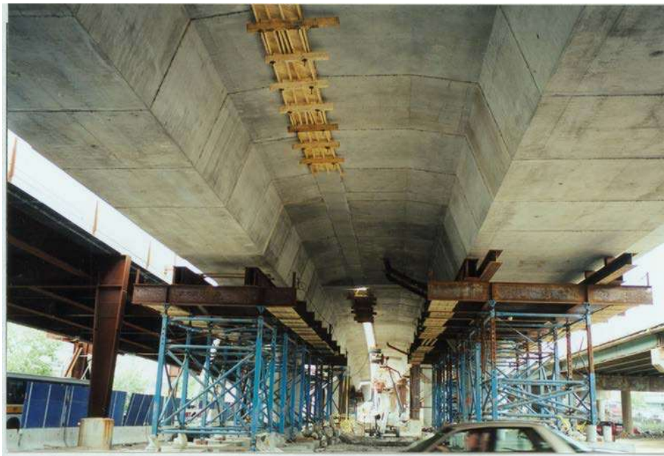
Figure 9.11.13 Adjacent Single Cell Boxes with Closure Pour
