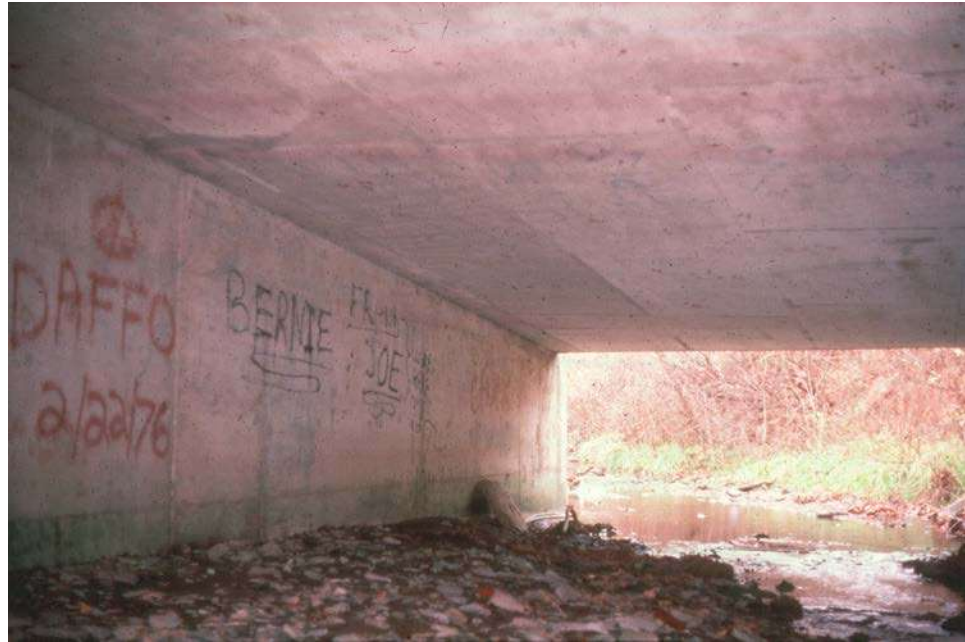
Figure 9.1.4 Bearing Area: Cast-in-Place Slab
