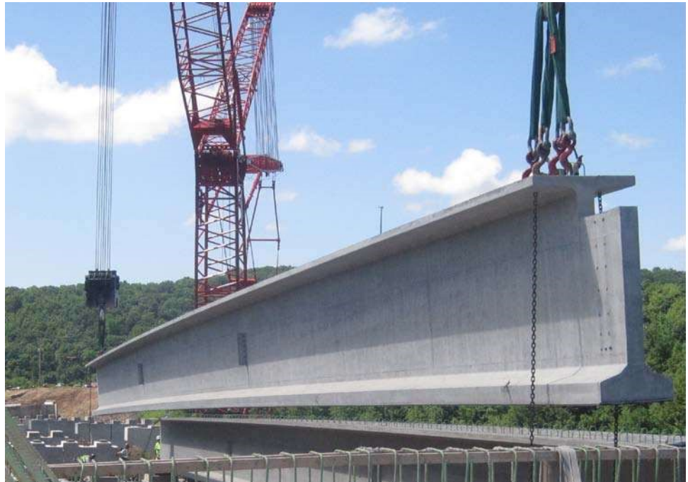
Figure 9.9.5 Placement of an AASHTO-PCI Bulb-Tee Beam
