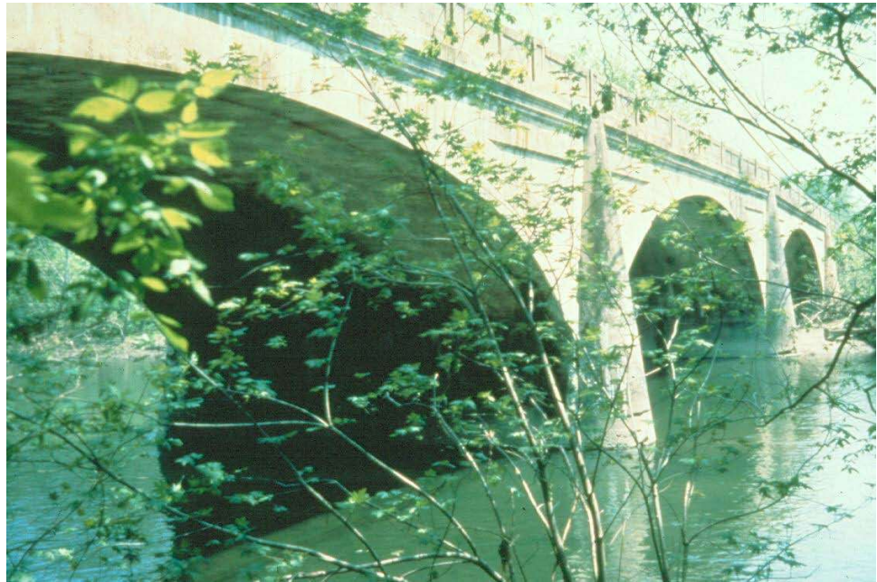
Figure 9.5.2 Multi-span Closed Spandrel Arch Bridge
