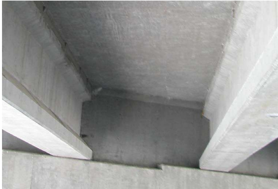
Figure 9.9.15 Bearing Area of a Typical Prestressed I-beam
