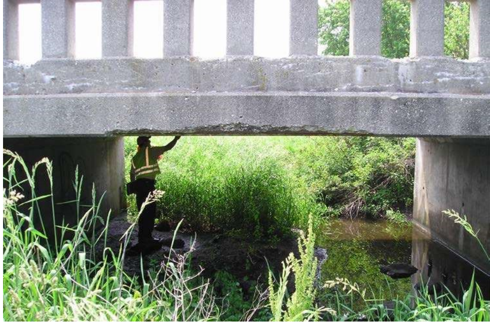
Figure 9.1.7 Inspector examining and documenting deficiencies in concrete slab
