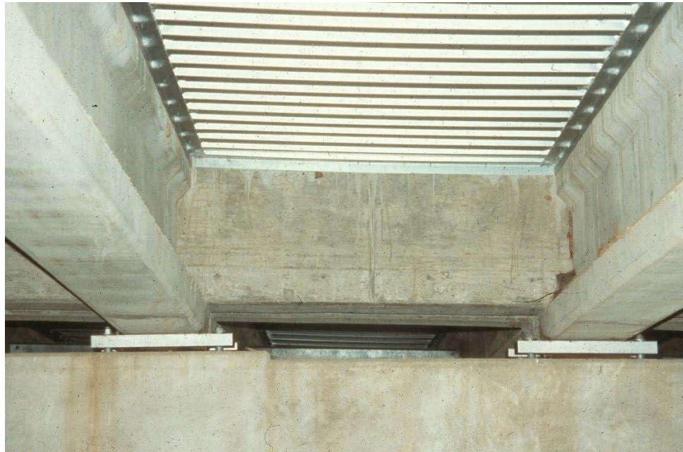
Figure 9.9.18 Concrete End Diaphragm
