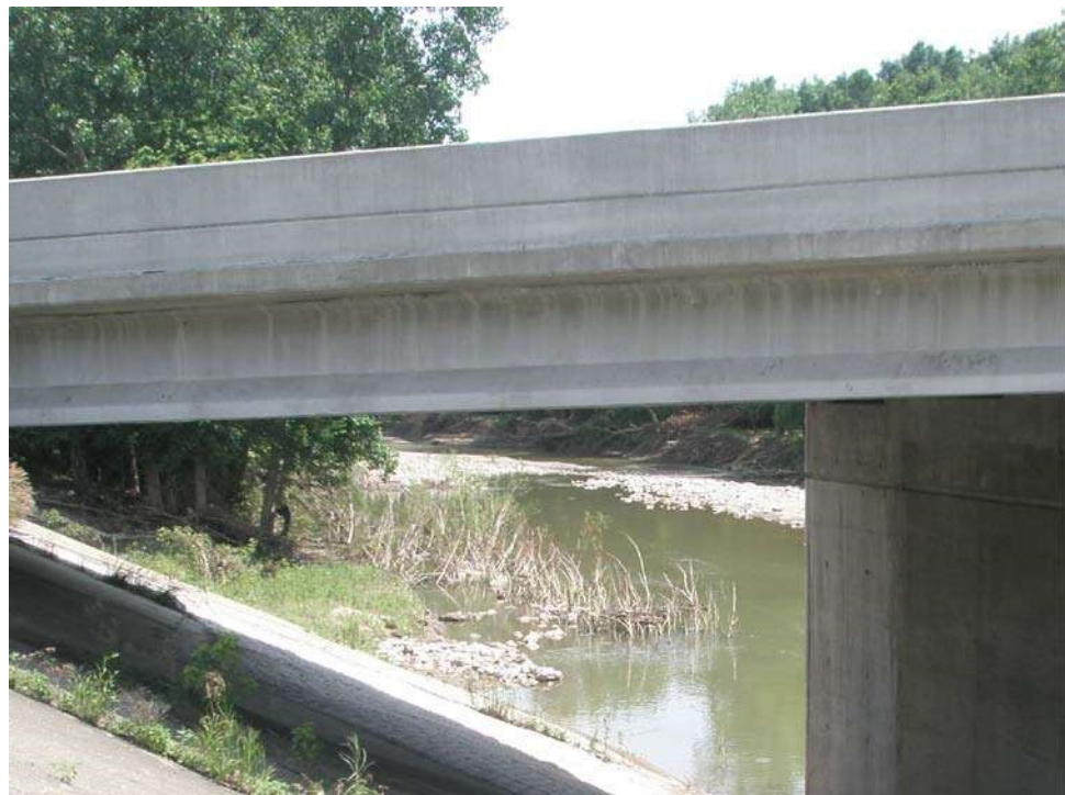
Figure 9.9.3 AASHTO Prestressed I-beam Bridge
