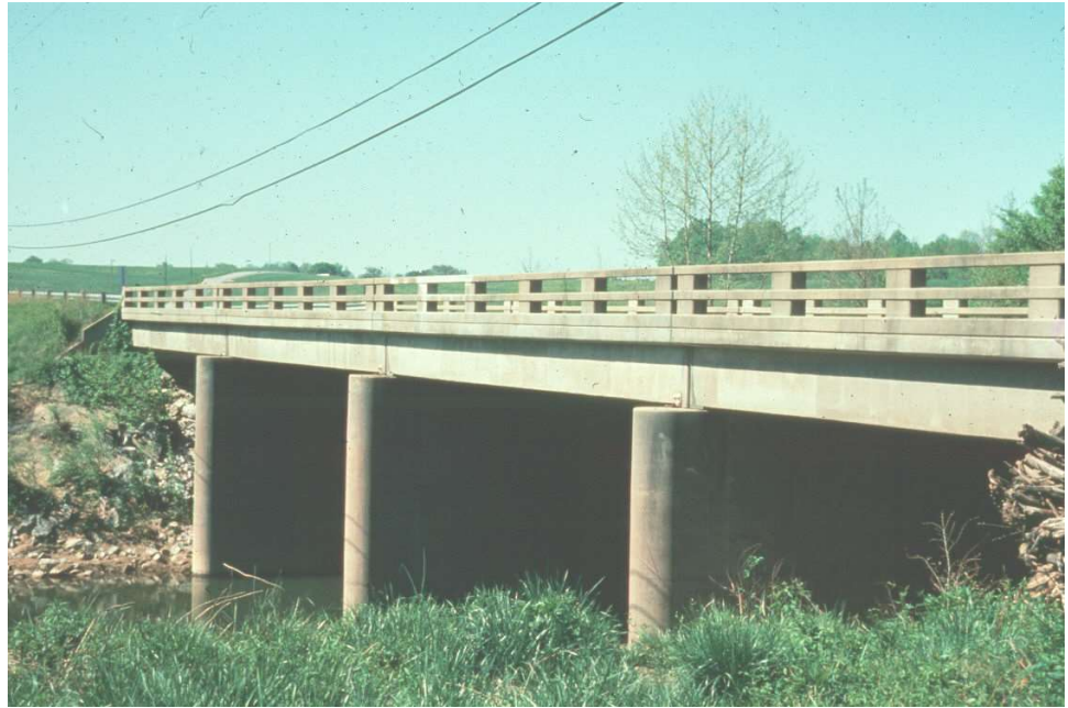
Figure 9.10.1 Typical Box Beam Bridge
