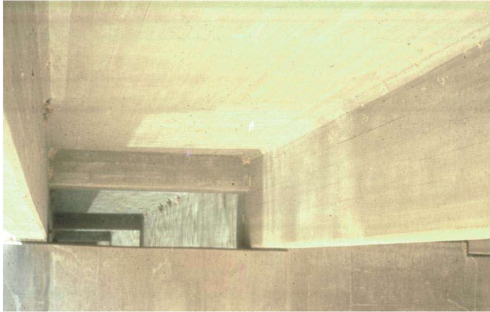
Figure 9.2.6 Tee Beam Primary and Secondary Members
