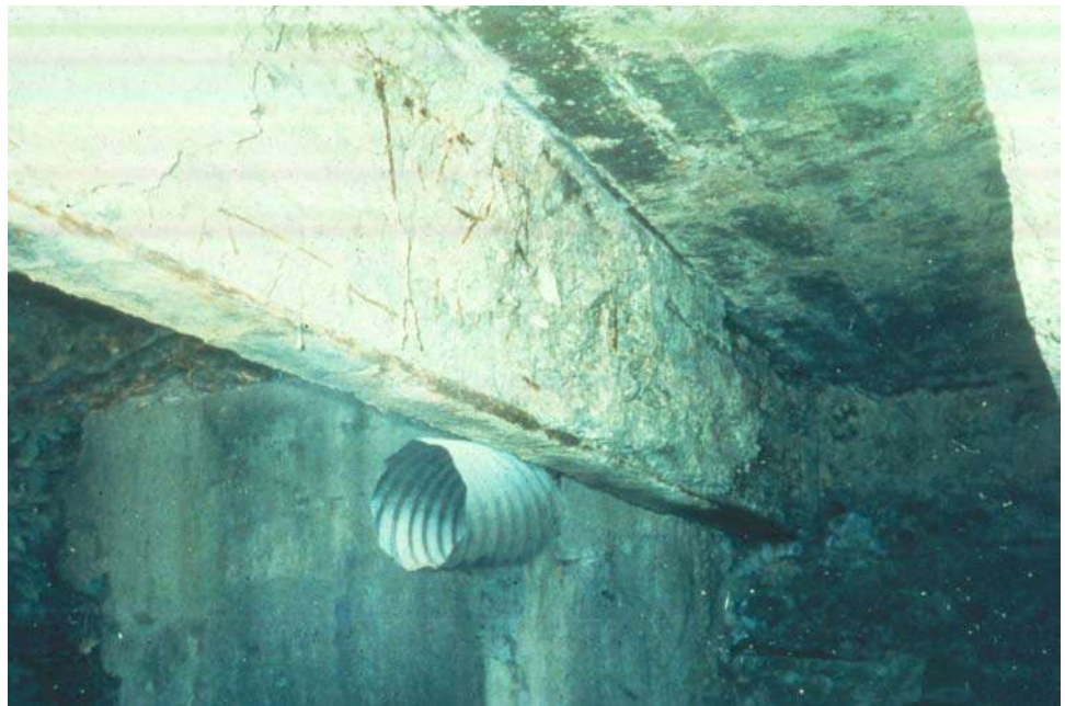
Figure 9.2.5 Concrete Encased Steel I-beam
