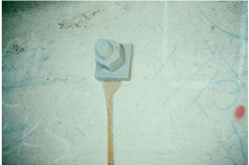
Figure 9.4.8 Close-up of Stem Tie-Bolt (Epoxy Resin)
