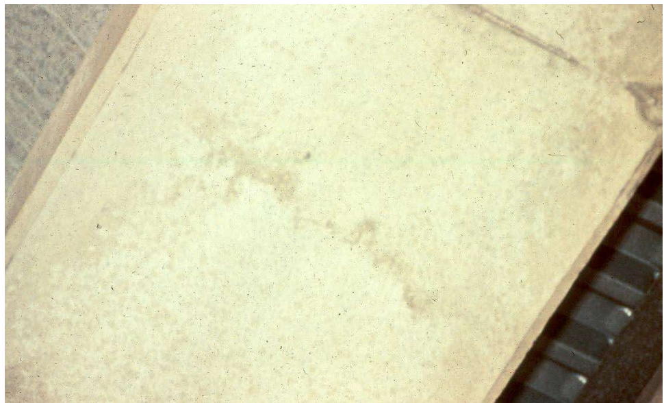
Figure 9.9.17 Flexure Crack
