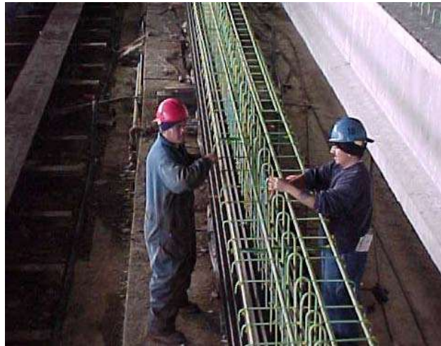
Figure 9.9.11 Extended Stirrups to Obtain Composite Action
