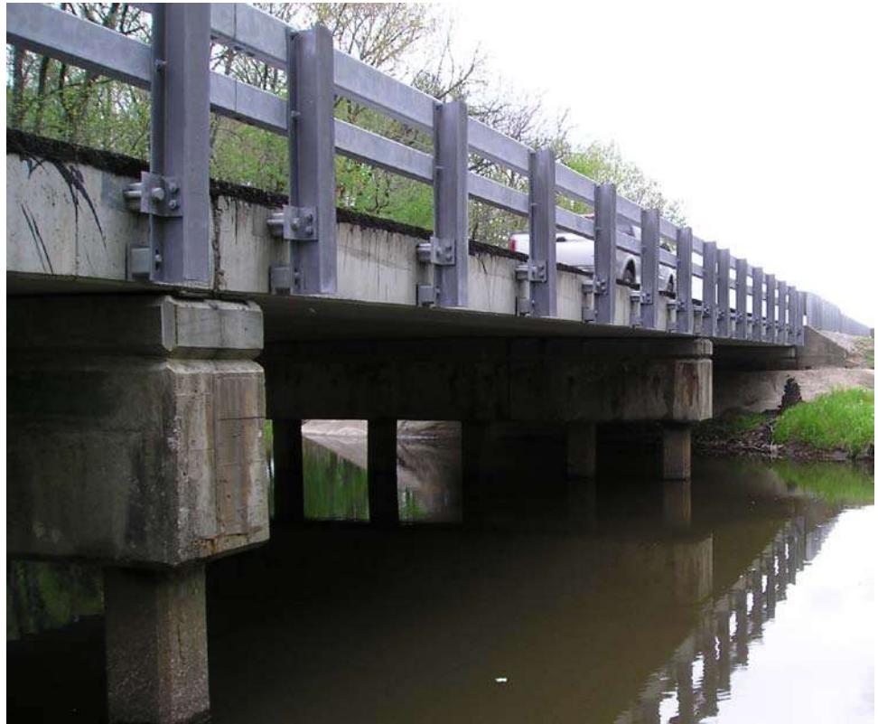
Figure 9.7.1 Typical Prestressed Slab Beam Bridge
