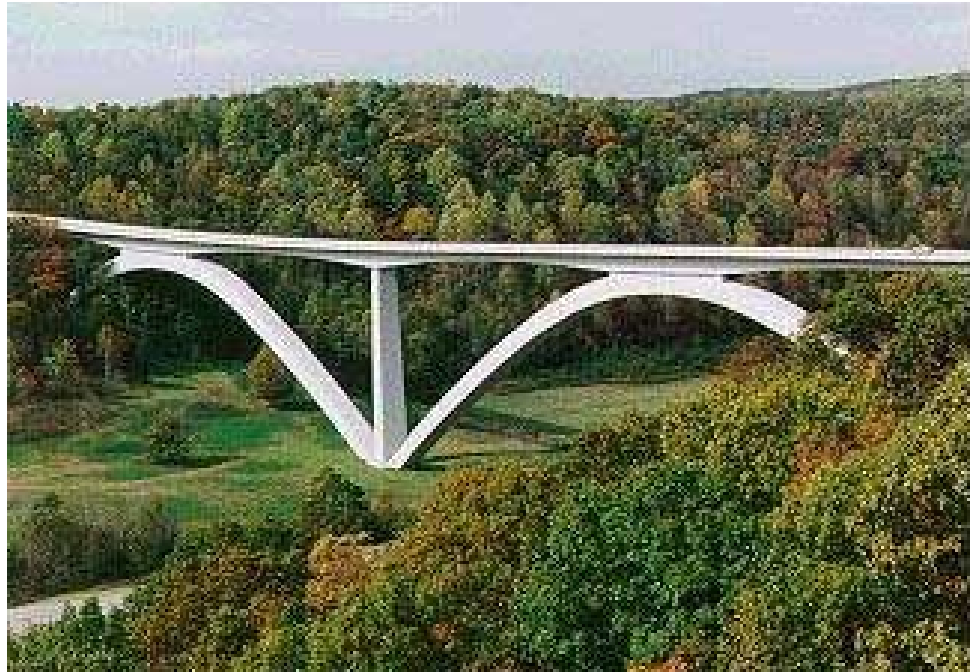
Figure 9.5.6 Precast Post-tensioned Concrete Arch without Spandrel Columns
